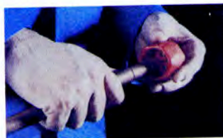
Removing the burrs with a reamer
